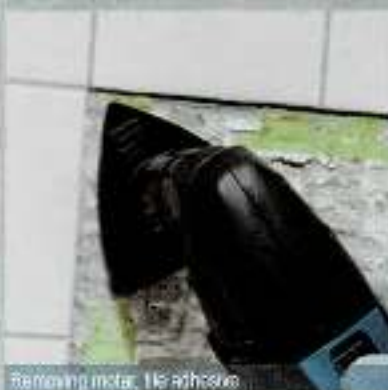
Removing metal tile adhesive
