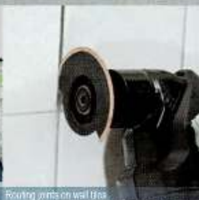
Routing joints on wall tiles
